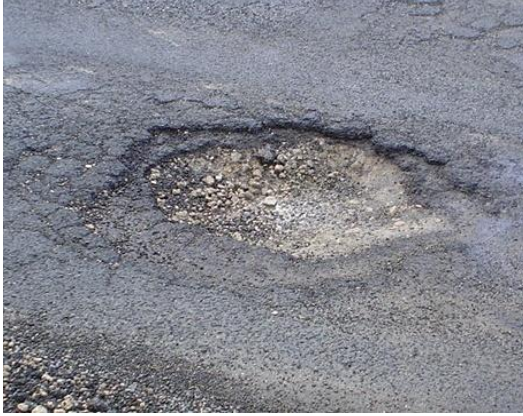
Fig.1.4 potholes
