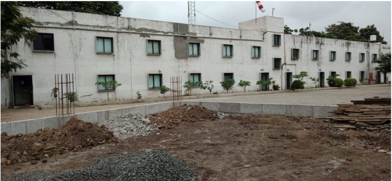
Fig. 1 – Front Elevation of Industrial Building
